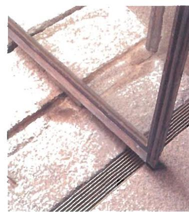
Pivot door and threshold providing drainage and threshold transition
