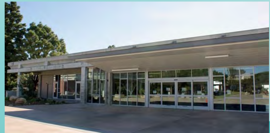
Student Affairs Building ("M" Building) Renovation
