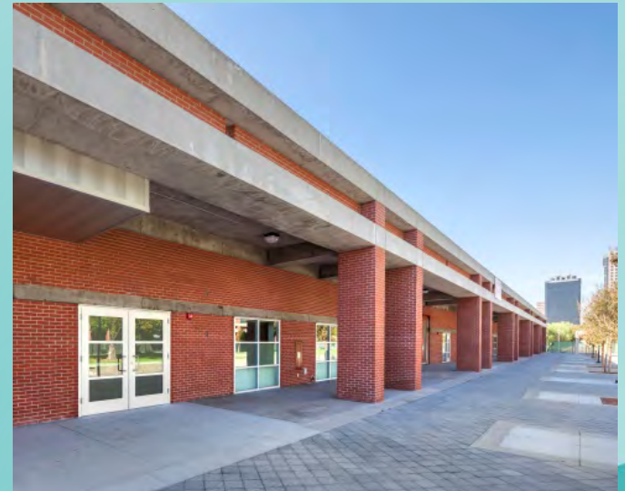
"C" Building Renovation
