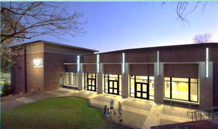
Arts & Humanities ("H") Building
