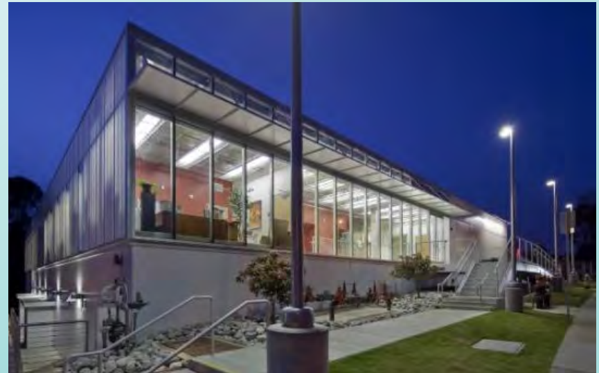
Health, Exercise Science and Athletics ("P" Building) Renovation
