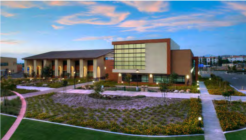
Business & Math ("M") Building
