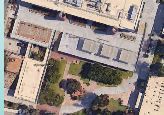
“D” Building roof courtyard
