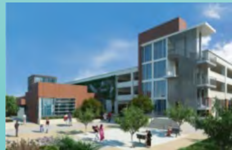
Miramar College Police Station
